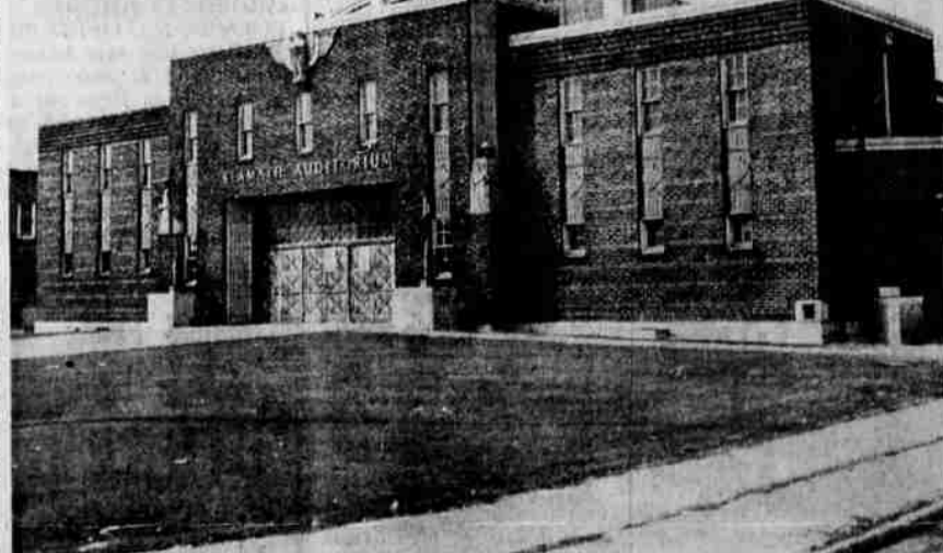
THIS BUILDING would become a new Civic Recreation Center under provisions of a proposal presented to the city council last night by Park and Recreation Director George Price. The proposal is subject to approval of the Armory Board and financial participation of both the city and the county. The council indicated its willingness to take part in the program Monday night. Price would increase use of the building, both for space rentals as well as recreation and other uses. The Klamath Auditorium was built a number of years ago, financed by both the city and the county and is operated by an Armory Board appointed by both groups.
