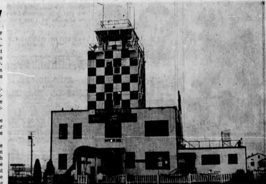
TAGGED FOR DESTRUCTION is this obsolete terminal building at the municipal airport. Constructed during World War II, the building has proved inadequate to serve the expanding needs of the air service into Klamath Falls. The Gospel Mission has undertaken the task of tearing down the old building to clear the area for the new terminal nearing completion behind this tower. The structure should be razed within 60 days.
