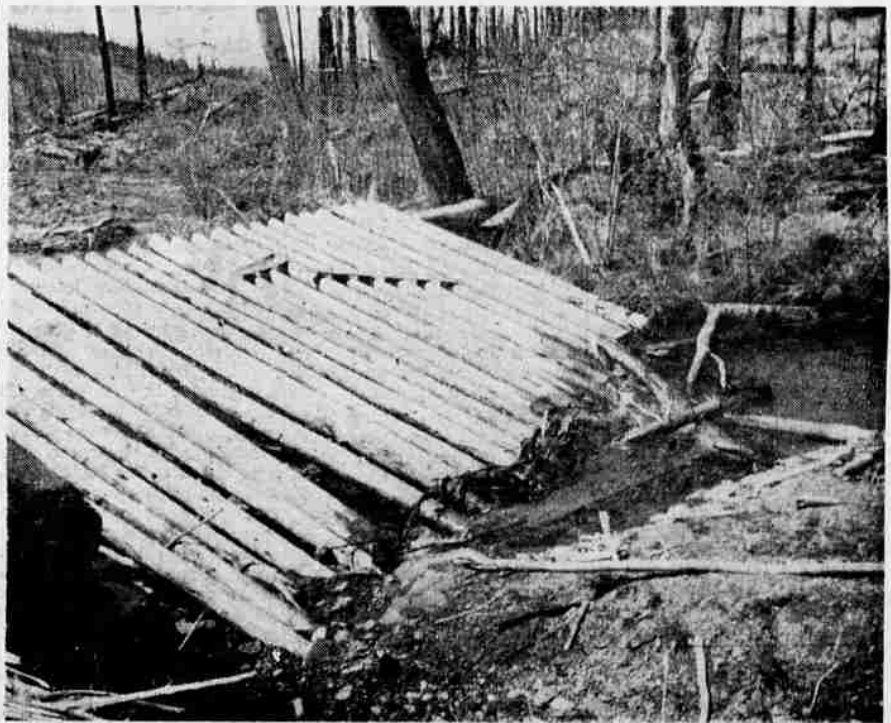
TRASH CATCHERS such as this one have been installed in the drains in the Deming Creek burn area to allow free runoff and prevent plugging during heavy runoff periods. This is one of the many items studied by last summer's show-me tour of the Deming area. — Photo by McGee
