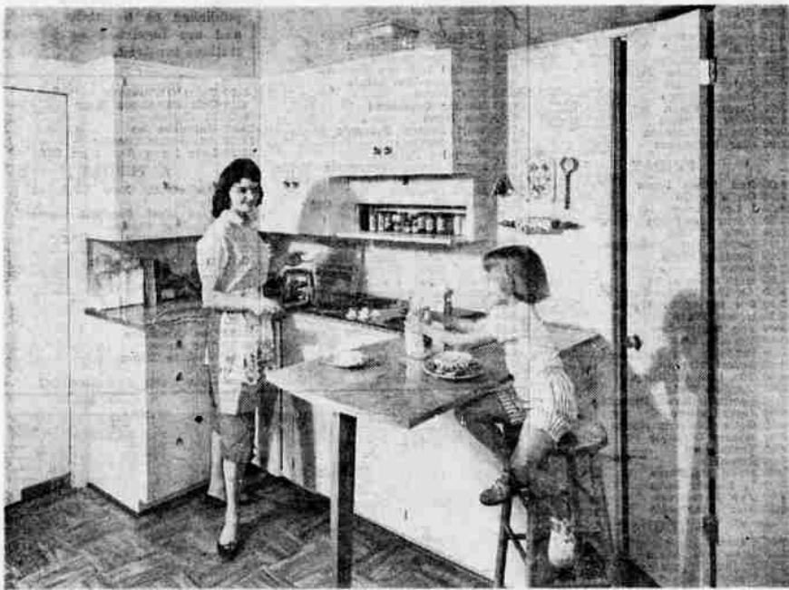
SPACIOUSNESS A RESULT OF PLANNING — Corner of this petite, but handy, kitchen illustrates that spaciousness is not always a matter of size. Excellent planning is evidenced here by convenient placement of cabinets, use of built-in range, and a work counter which doubles as a breakfast bar. Cabinetry was executed in durable Douglas fir lumber, painted a cheery pastel shade.
