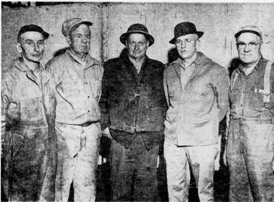
PLANT EMPLOYEES still on the staff who were present for the December 16, 1929, opening of Weyerhaeuser's big pine mill on the Klamath River include, left to right, Jim Stafford, machine shop; Richard Griffith, blacksmith; Bill Crawford, pond foreman; Ralph Williams, box factory foreman and Jim Hunter, machine shop foreman.
