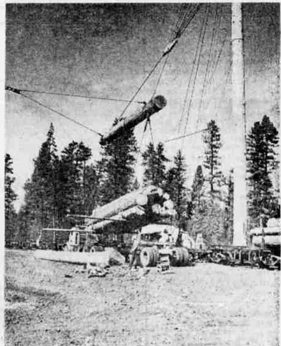
THEN AND NOW: Loading logs on a flatcar with the use of a jammer as shown in the top picture by Ted Durment, was a far cry from the modern truck haul and reload with gas powered equipment, as shown in the lower picture taken by Eugene Gjertsen in September of this year. Durment remembers taking the top picture but couldn't recall just when it was snapped. Notice the absence of hard hats on the hook men and the loader. Both operations pictured are those of Weyerhaeuser Company which celebrated its 30th anniversary in Klamath Falls on last Wednesday.
