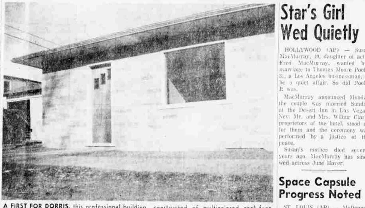
A FIRST FOR DORRIS, this professional building, constructed of multicolored rock-face tile, has been completed.
