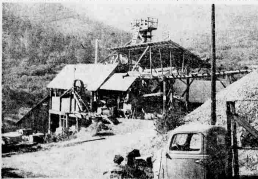
THIS BUILDING houses all the complex machinery of the dry-ore concentrator under the same roof. The concentrator is located in the lower left hand corner of the building. Elsewhere are the ball mill that grinds up the ore-bearing rock, the various big diesel motors and the other equipment necessary to the process. — Photo by Dow
