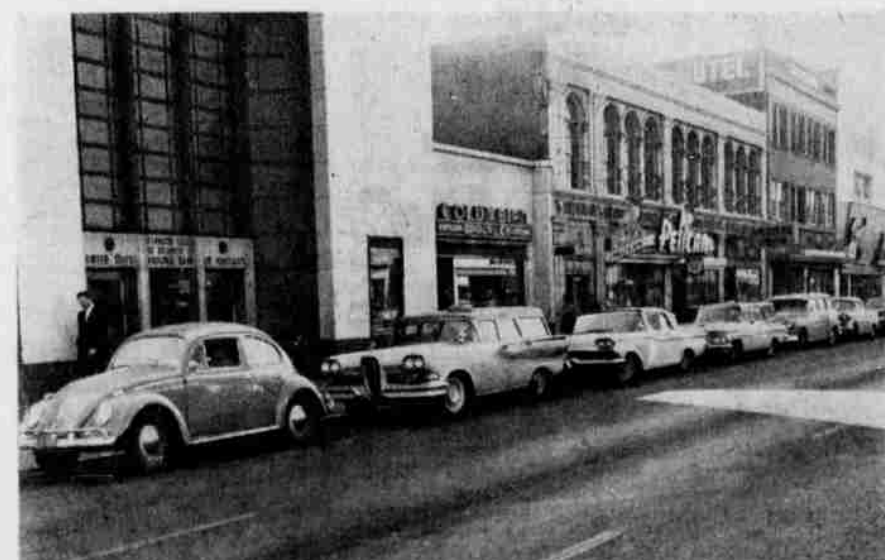
THE NEW TANDEM PARKING system is being installed on Main Street from Fourth to Eleventh. These three pictures illustrate the change in parking that the new system will affect. Far left is a picture of the old style, front and spaced parking, where each car has a few feet in front and a few
