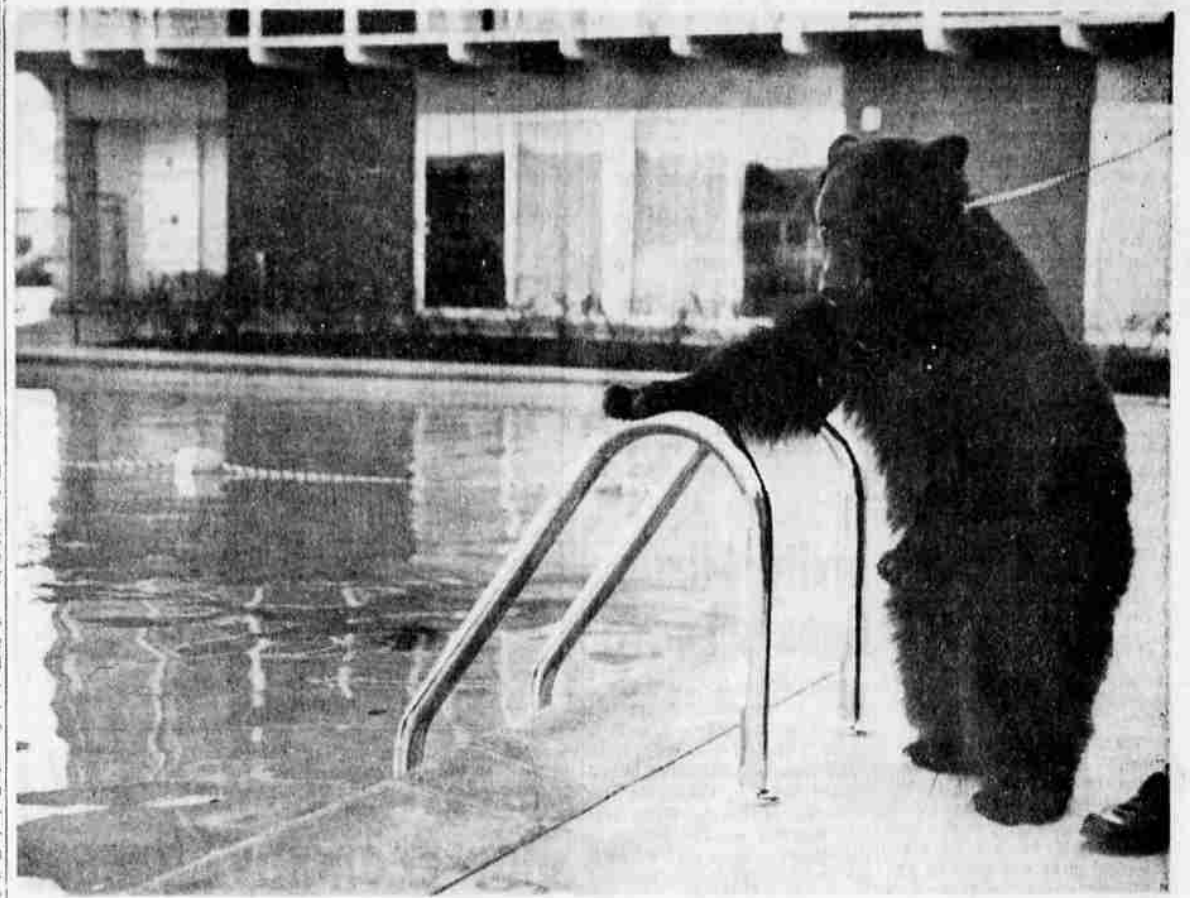
THE WATER IN THE NEW SWIMMING POOL at the nearly completed Rickfalls Apartments looked awfully cold to the little Moore Park bear the other day when he paid a visit to the construction site. The bear, name to be announced soon as the result of a citywide contest, was probably out looking over the new apartment building to see if he could get any ideas that would apply to his new quarters. Contributions are now being accepted by George Price, city parks and recreation director, toward a fund for constructing a new bear pen at the city park. About $200 has come in to date toward a goal of $1,000. Those wishing to contribute may send their check to Price at city hall. The pool shown here lies behind the completed office unit at the new apartment with four studio apartments on the top deck.
