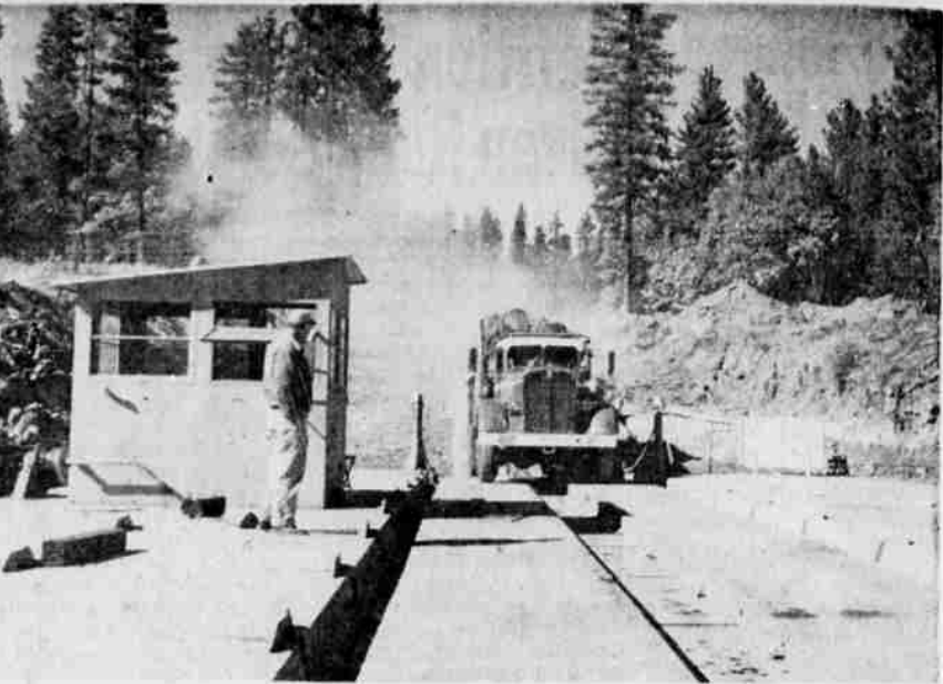
A LOADED TRUCK drives onto the Lake Britton Ferry. The Lorenz Company at Burney has devised this unusual method of transporting logging trucks to its big mill. Since the company owns its own roads leading to and from the ferry, trucks may be loaded to their capacity without fear of being in violation of highway load limits. — Photo by McKinney
