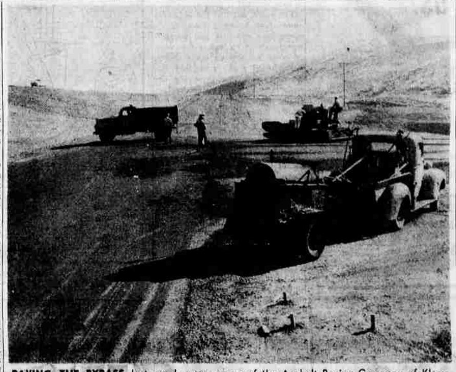
PAVING THE BYPASS last week were crews of the Asphalt Paving Company of Klamath Falls. Work is nearly complete and the fast stretch should be open for traffic in about a month, barring delays.
