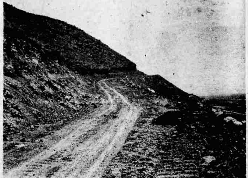
DOHERTY SLIDE proved one of the toughest sections of the Adel-Winnemucca road to construct because it was a straight dynamiting job for about three miles. The only rougher portion of the road constructionwise is anticipated to be Greaser Canyon. — Photo by McKinney and Bennett
