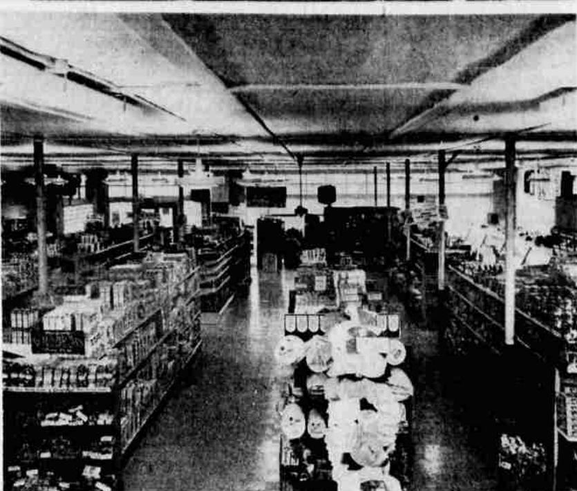
NEWLY REMODELED interior of the Market Basket, Ninth and Pine, is shown in this photo. Selling area was extended at the rear of the store by taking in former warehouse space. This makes possible wider aisles and enlarged produce section. Remodeling was done by Warren Parr, and the grand reopening was launched Thursday by Dick Hicks and Norm Duffy, co-owners of the store.
