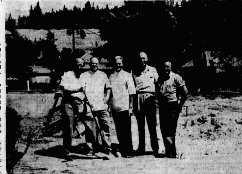
A MEDICAL-DENTAL BUILDING will rise where these men turned the first spadeful of dirt in Weed Thursday. From left they are Dr. H. L. Vidricksen, a physician; Dr. L. L. Johnson, a dentist; V. J. Thompson, M. D.; James Mallory, president of Weed Chamber of Commerce, and Joe Quadros, contractor who will build the plant.
