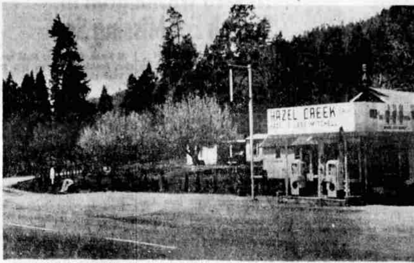
HAZEL CREEK STATION, 10 miles south of Dunsmuir, was the site of an early-day hotel and coach stop connecting California and Oregon settlements. It will soon be demolished to make room for the last part of the freeway being built near Dunsmuir. The picture plainly shows the ancient cherry trees extolled by Mark Twain who stopped at the hotel when he was traveling with Gen. U. S. Grant.
