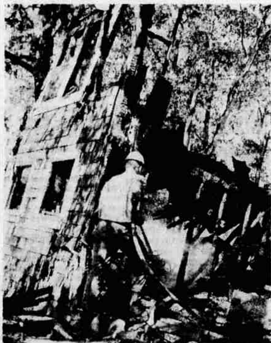
DIRK CHANDLER, Castella, a member of the U. S. Forest Service fire suppression crew, carefully checks the wreckage of the fire-damaged home of Mrs. Mable Benkosky in Dunsuir. Extremely dry, hot weather makes any blaze a menace to the entire area, Paul Dryden, fire control assistant, explained. Mrs. Benkosky suffered second degree burns and shock when her home was destroyed early Saturday morning.
