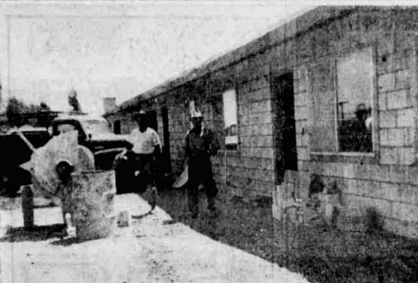
FIRST NEW HOUSES to be built in Bly in many years are nearing completion. Across the street from the mill site, the houses are punice brick with red cinder roofs. Built by the Bly Lumber Company, the homes will be occupied early in August by the F. E. McGee and D. L. McGee families. Paul Buck, contractor from Klamath Falls, is shown, right, with his helper, William Robinson. —Photo by Roberta McGee
