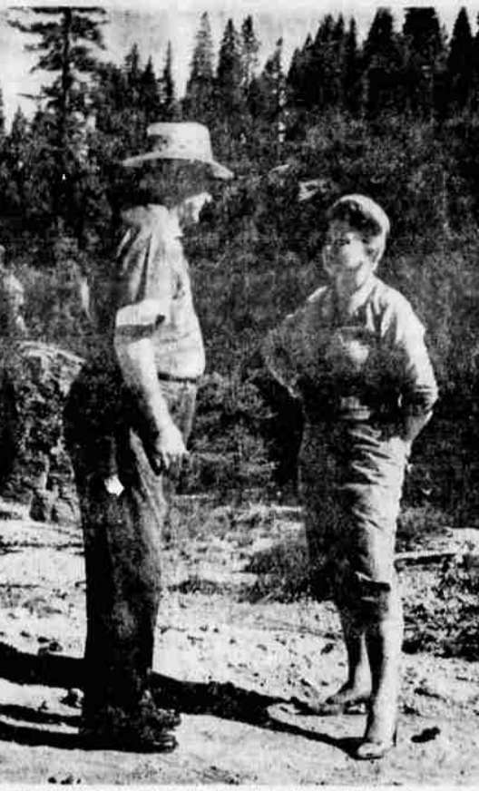
MRS. PAULINE DAVIS (D-Portola), Second District assemblywoman, with Siskiyou County Supervisor Art Barr inspects proposed Box Canyon dam site. Box Canyon is on the Sacramento River five miles southwest of Mount Shasta.
