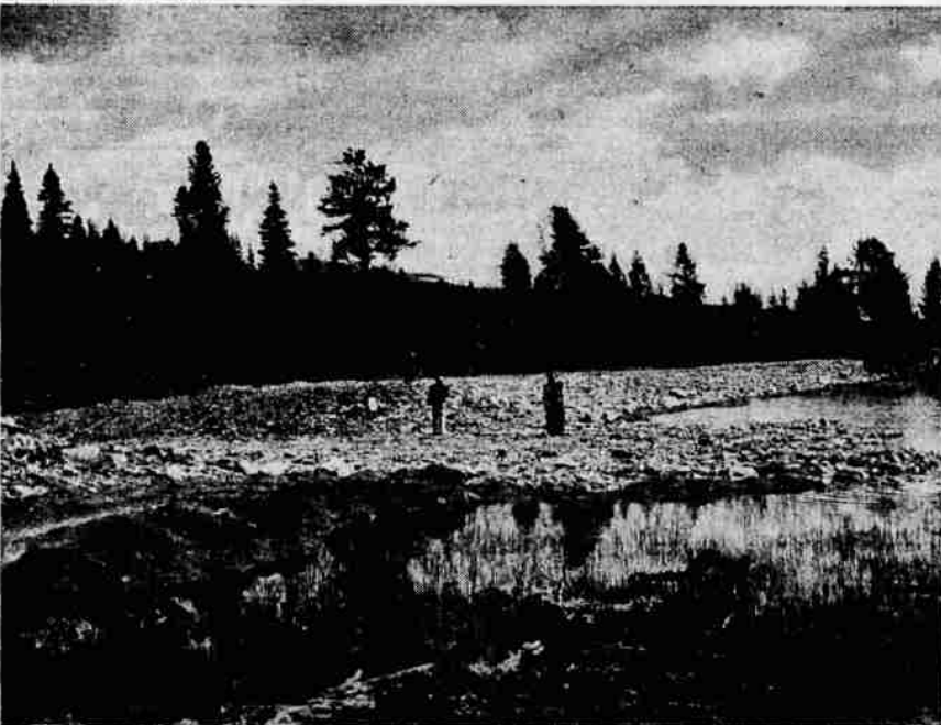
THE PERMANENT SPILLWAY of the forest service dam at Lake of the Woods is seen here. When the lake reaches its maximum level the water flows off through this rock-lined channel into proper drainage canals. Since installation of the dam a good deal of the flooding trouble around the lake's airstrip has been overcome.
