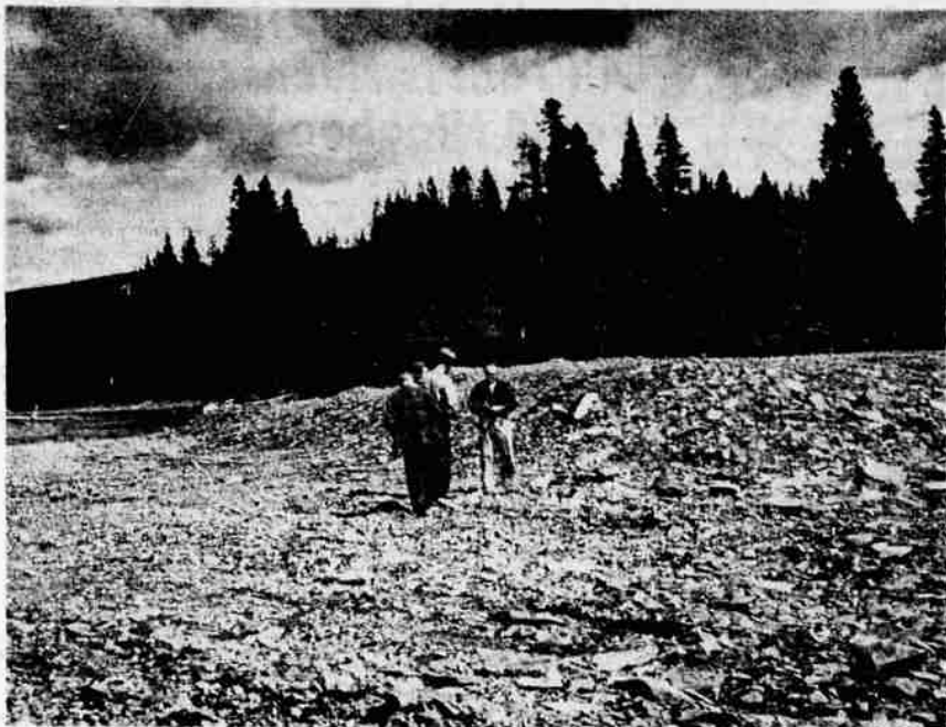
THIS LOW DAM at Lake of the Woods was completed by the U.S. Forest Service last year. Purpose of the structure is to maintain the level of the lake and the control runoff by diverting it into a standard channel. Located opposite the airstrip the dam has served the intended purpose well, according to forest service officials. At the left of the picture can be seen the spillway which leads to the drain. No gates or other moving equipment are necessary with the dam.
