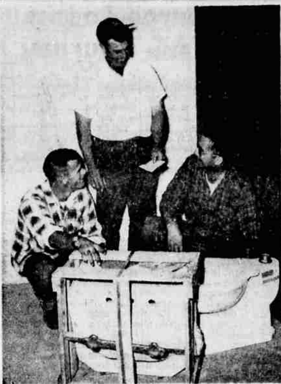
PLUMBERS IN THE ACT — As the Mills Little League Ball Park rapidly nears completion, Klamath Falls plumbers, Roger Wiseman, left, Art Stites, center, and Eddy Morlan, right, volunteer their services in installing plumbing in newly constructed rest rooms. The city park and recreation department, under the direction of Roy Harris, is currently giving the diamonds a thorough going-over in preparation for opening day.
