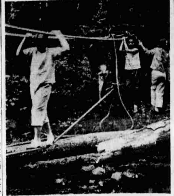
CONSTRUCTING a primitive rope bridge across a stream are these Girl Scouts, at the recently held day camp of the southern Siskiyou District of the Sierra Council. Other skills learned were how to prepare a three-course outdoor meal, how to make a "dribble can" for washing and how to recognize nettles and other woods hazards. Camp was established by dividing the Brownies and Girl Scouts into small units, each of which evaluated a site and made camp with sanitary provisions, rest and work areas and campfire and cooking areas. The camp was restored to its natural appearance at the close of the period.
