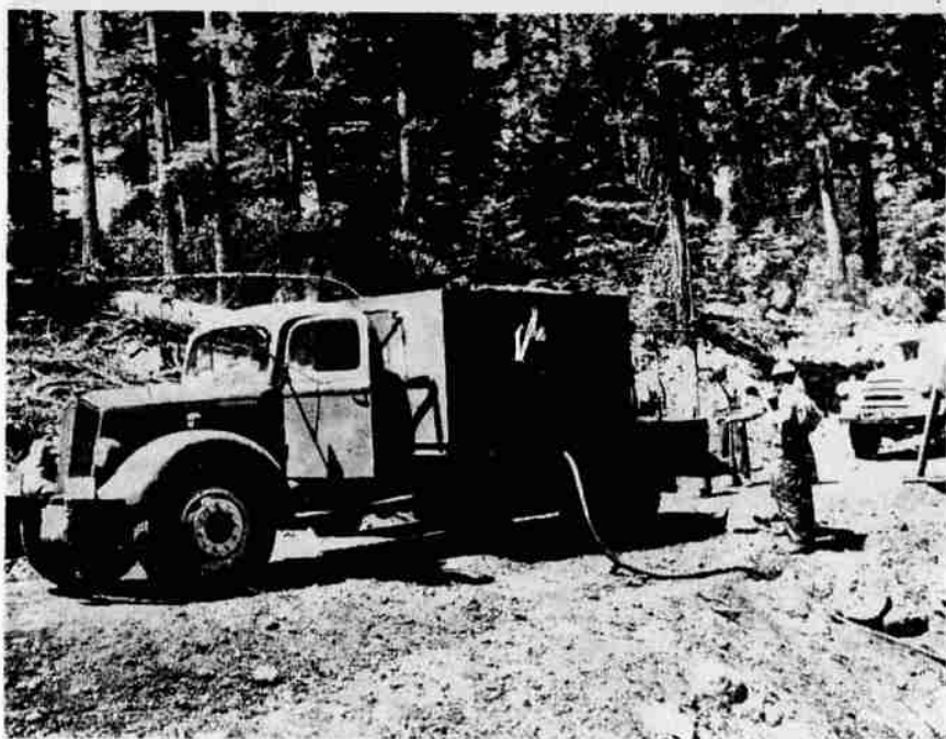
THE TANK CAN BE FILLED from any roadside supply on this combination sprayer and fire suppression rig developed by KPFA and WTC. The rig is shown here being filled at Grub Spring west of Klamath Falls. The truck can be used in fire suppression work and as an alternate water supply for fire tankers where necessary. This spring the truck was used for the first time in killing roadside brush by spraying. It is currently on standby for fire control duty.
