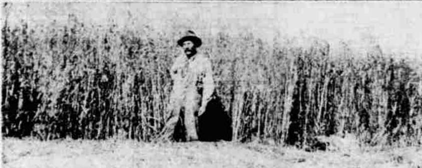
HAND-PEELED POLES were used in the construction of this barn at the Hagelstein ranch at Algoma. It was built 60 years ago by George Hagelstein and his father, the late John Hagelstein who is pictured in the lower photograph standing in one of the fields during grain harvest. The barn is still in use on the ranch which was homesteaded in 1894.
