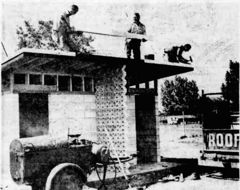
BUILT TO LAST — Fitzgerald Roofing tackled the job of putting the roof on the new restrooms at Mills Little League Park Saturday and when they did they put one on to stay. Shown in the process of applying a built-up gravel roof, guaranteed for 20 years, are Cecil Fitzgerald, left, Dan Taylor, center, and Dave Watson at right. Volunteer workers, they hope to be joined by parents and players in putting on the finishing touches to the new ball diamonds.
