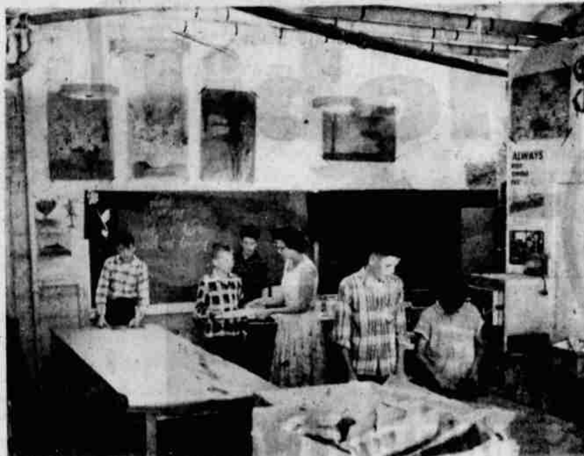
ORIGINALLY A STORAGE ROOM, the art classroom in the Dunsmuir Elementary School has a noise problem because of exposed plumbing pipes. —Photo by Don Kettler
