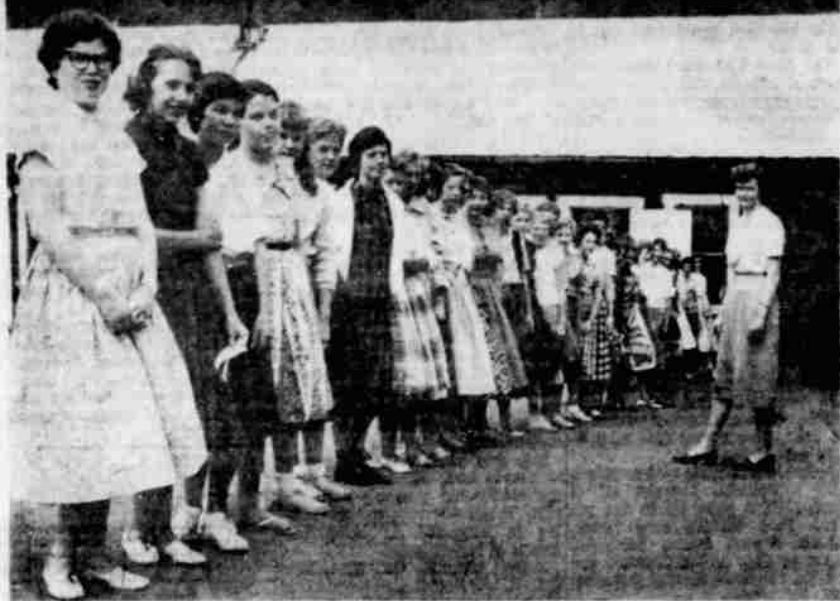
LINED UP outside of the condemned frame building of the Dunsmuir Elementary School is the chorus class which meets there. At a recent meeting of the school board, no decision was made as to the remodeling of the building. Time is important in the remodeling as it is hoped to have it ready by the fall term. It is considered unfit for pupil use because of fire and safety hazards. —Photo by Don Kettler
