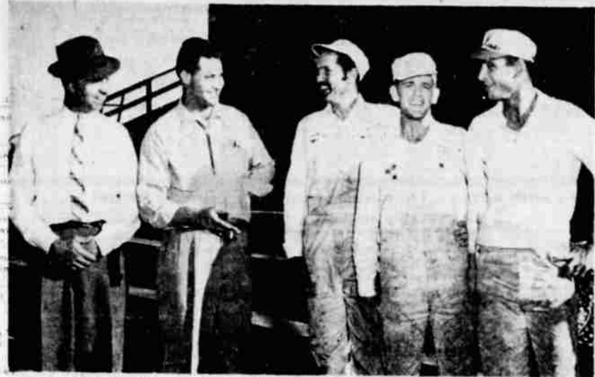
BALL PARK PAINTING - A SPECIALTY — KC Painters, with an assist from the General Paint Company, tackled the paint-thirsty Mills Little League Park bleachers with a vengeance Thursday to give the project a big boost. Volunteering their services at the end of their regular work day, Keith Coddington's KC Paint crew poured 35 gallons of paint onto the greasy rebuilt bleachers, then had to send out for more paint. M. E. Mountain, at left, Portland representative of General Paint obliged, readily. Pictured, from left to right, Mountain, Keith Coddington, Ed GeRue, Wayne Bryan and Richard Blavins.
