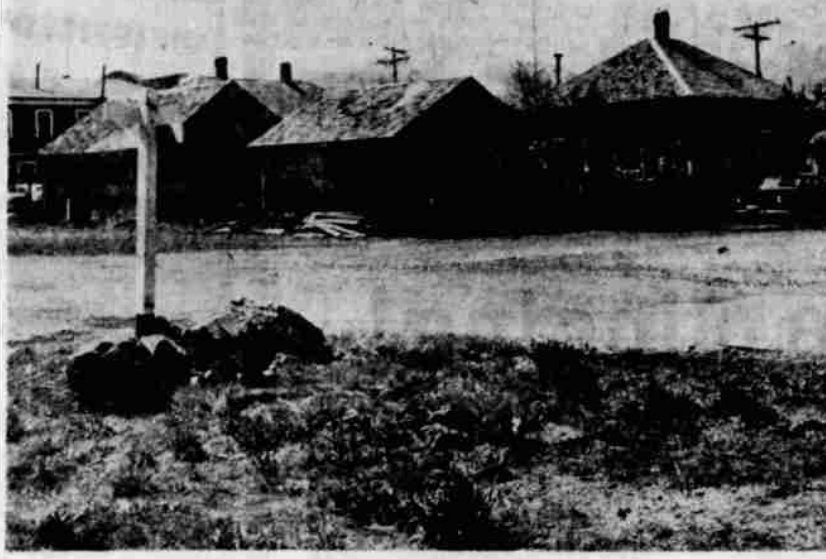
MOVING DAY IN WEED saw these two houses recently moved from Main Street to two different sites on Gilman Avenue. The International Paper Company, Weed Branch, is owner of all of the property concerned. The Main Street site is being cleared for possible future business developments.
