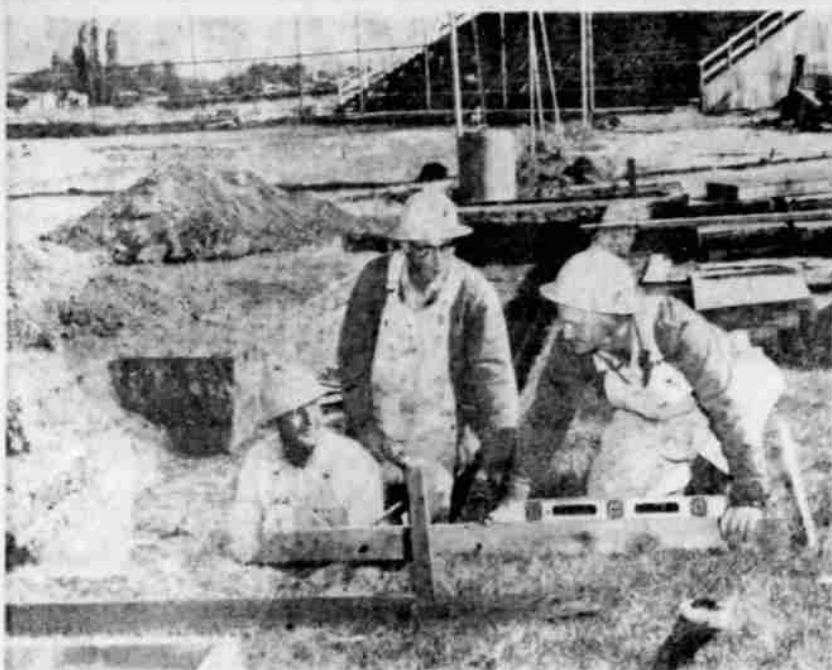
MILLS LITTLE LEAGUE PARK —More volunteer workmen swung into action on the new home for Klamath Falls Little Leaguers when the Vik Construction Company, represented by Jim Hall, left, Herman Westlund, center, and Red Williams, right, tackled the job of building the forms for concrete bases of the intended dugouts. The Vik crew was joined by Pacific Telephone Company workers who voluntarily set up the posts for the backstops and approximately 55 Little Leaguers and fathers, all pitching in to speed the work on the park.
