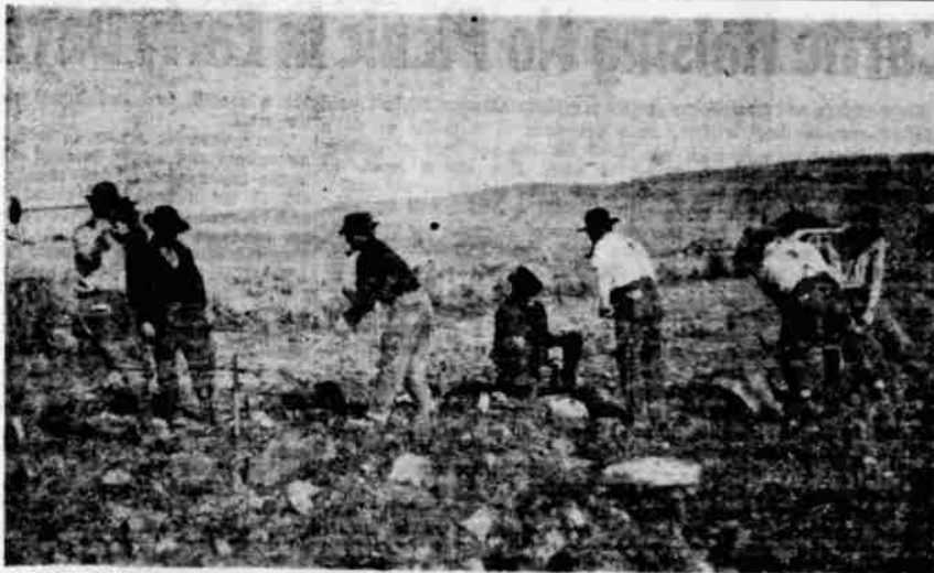
HAND TOOLS and many hours of work went into the enlarging of the old Adams Canal, now the "A" Canal north of Malin that carried irrigation water in 1910 to land in the southern part of the Klamath Basin. Far left, facing camera, is William Halousek, one of two of the original settlers still living in Malin. Others are unidentified.
