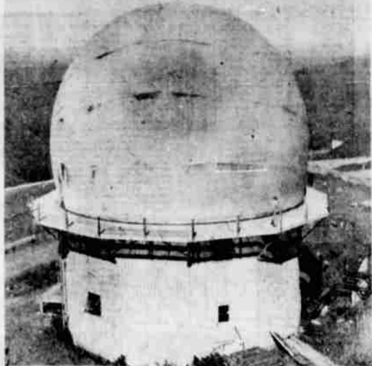
THIS IS one of three radar domes atop Haymaker Mountain above Keno housing giant telescope-like radar scanners that reach far out to sea. The entire dome above the walkway is supported only by air pressure.
