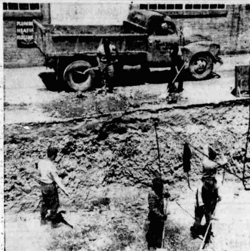
THIS EXCAVATION is the start of a three-story addition to the Klamath Falls Gospel Mission. All work to date has been done by men who have visited the mission, received help and volunteered their labor. Truck in background was donated by Kenneth Nelson, excavation contractor for removing dirt dug by hand with pick and shovel.
