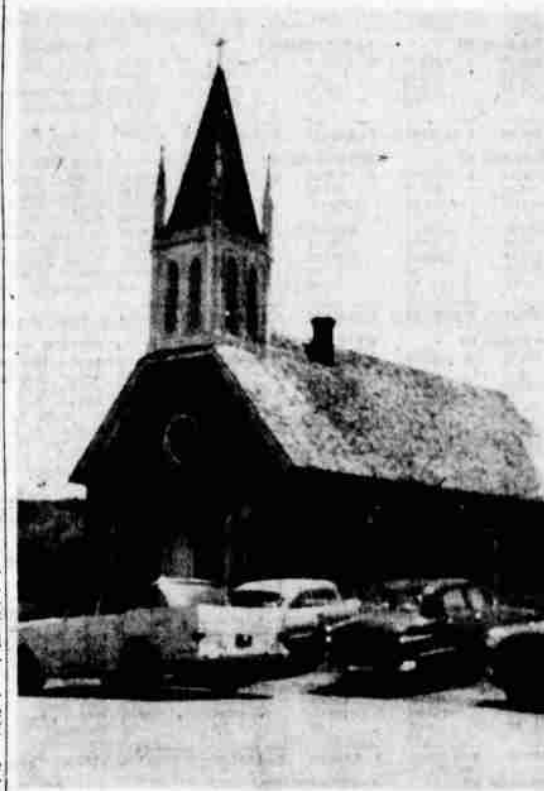
THE OLD Hawkinsville Church, now open only to the large Portuguese congregation on the Feast of the Holy Ghosts and the Immaculate Conception, is said to have been converted from a brick building that had housed a saloon and general merchandise store, erected in 1858 at the time when Hawkinsville, now a ghost town, had 2,000 inhabitants. The building was converted into the edifice as it stands today about 1870 when a Father Farrelly turned his attention to the Hawkinsville Catholics and established the parish.
