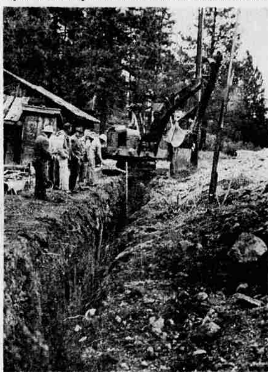
THE LAYING OF SEWER LINE in West Chiloquin is just about finished. Jeske Brothers Construction Company is doing the work. Shown here is a part of the crew inspecting the excavation work. The other sections of Chiloquin were completed earlier. Observing the work in the 12 foot trench are construction men and city officials. —Photo by Otto Ellis
