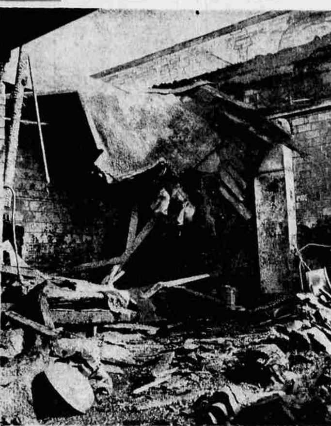
burning timbers in the front of the building in the photo at left. The picture at right shows an after-the-fire shot of the paint shop where the fire apparently started and where temperatures were hot enough to melt metal.
