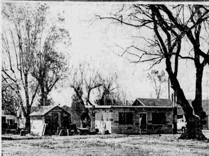
THE WIARD TRAILER COURT , opened by Mr. and Mrs. Harry Wiard, 2705 Wiard Street, is a new addition to the street named for the Wiard family. Building in the foreground of pumice tile contains laundry, showers and rest rooms. Trailer spaces are at rear of the building. The new court is close to the Wiard Park playground for children with picnic facilities for large groups as well as families. Mr. and Mrs. Wiard, in Klamath Falls for 33 years, at one time operated the Chicken Stile on South Sixth Street. Harry Wiard stands in front of building.
