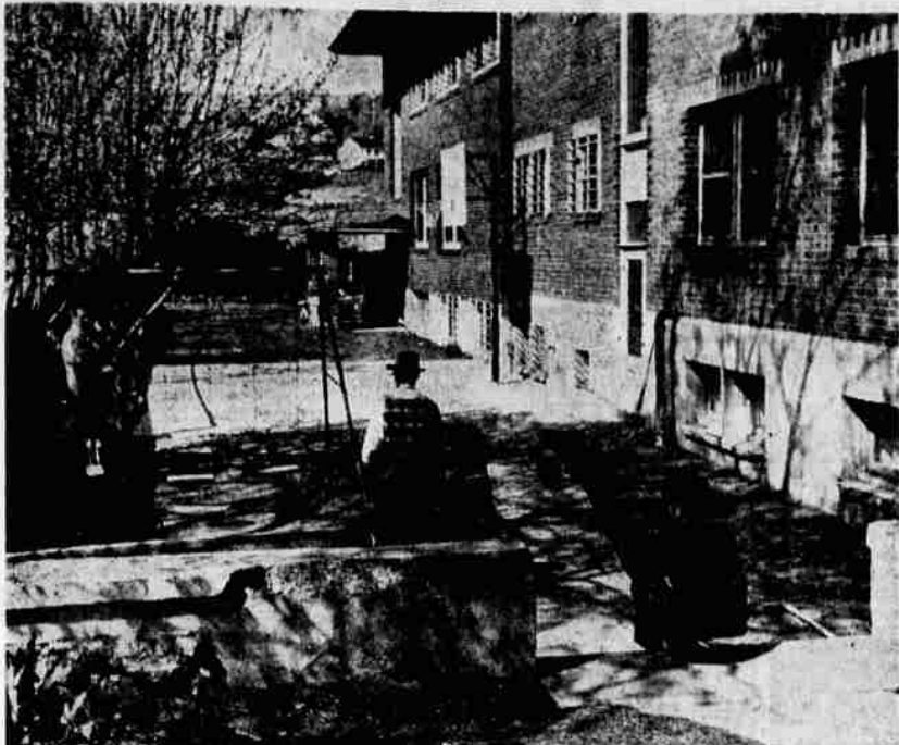
RECREATION SPACE is pitifully limited at the present juvenile home. This side yard is the only available area for boys and girls to get outside for supervised play. The basketball slab was constructed two years ago.
