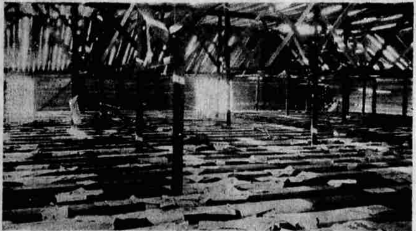
SUNLIGHT shone through the cracks in the roof of the building that went up in 24 hours to accommodate the crowd that came to hear Billy Sunday sell Liberty Bonds at the end of World War I in Klamath Falls.
