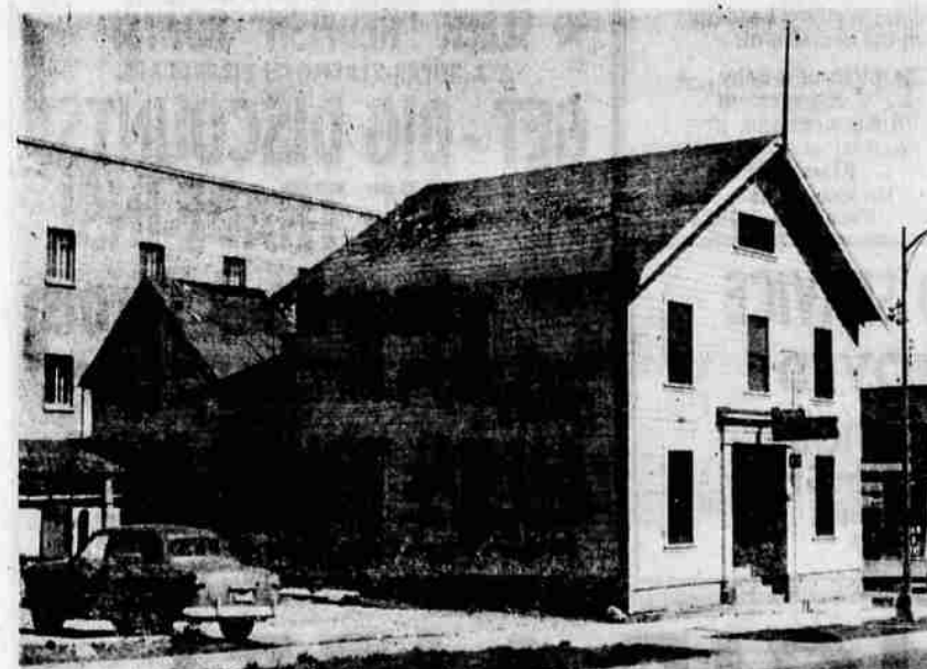
THE COLONIAL HOTEL on Eleventh Street between Main and Pine, is being destroyed by salvage men to make room for a parking lot that will handle 35 or 40 cars for the Winema Hotel. The Winema management has owned the building and site for many years. It has been operating until very recently. The Colonial was built before Winema co-owner Merle West came to town 45 years ago.
