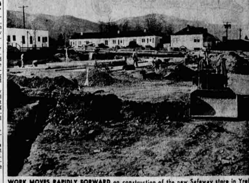
WORK MOVES RAPIDLY FORWARD on construction of the new Safeway store in Yreka. The modernistic store will feature over 12,000 square feet of floor space, and have parking capacity for 59 cars. Here, foundation work is well underway at the location at 729 South Broadway. The A. J. McMurray Company of Yreka is contractor for the work. Completion date is set for early summer for the building which will cost approximately $223,000.
