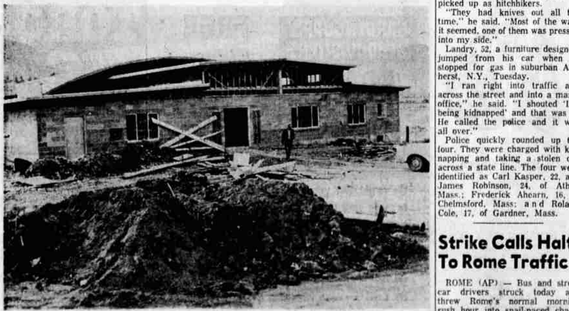
A 12 LANE BOWLING ALLEY nears completion in Yreka. Harry Millette will be owner and operator of the new business which is located just south of the city limits. The project will represent about a $200,000 investment. The building, shown here nearing completion, covers a floor space of about 10,000 square feet. There will be parking accommodations for 150 cars. The alley will feature automatic pinsetters.
