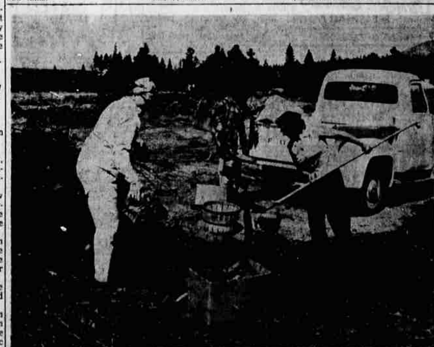
A WOMAN'S WORK is a mighty important feature in the clearing of the site for the College of the Siskiyous at Weed. Here Ethel Parkinson, Rita Renning and Mary Mazzell contribute their time and labor to assist in clearing debris from the site. They were among volunteers who have been working for the past two weeks to clear the junior college site. The Singleton Construction Company of Redding was awarded the contract for the three buildings at a bid of $101,967.
