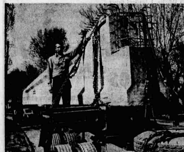
A UNIQUE SYSTEM OF TRANSPORTATION was used to bring these huge 105 foot long concrete beams from Portland to Klamath Falls for use in the California Avenue overpass. Far left, E. J. Sanderson stands alongside one
