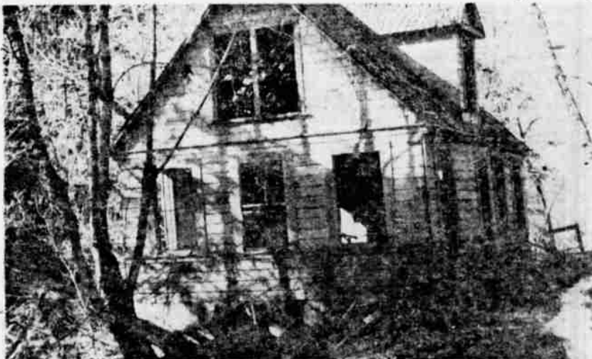
THE OLD DORMITORY was a busy place when Ney Springs was in its glory. Now all that remains is this battered wreck, blank windows staring out over the lush vegetation.
