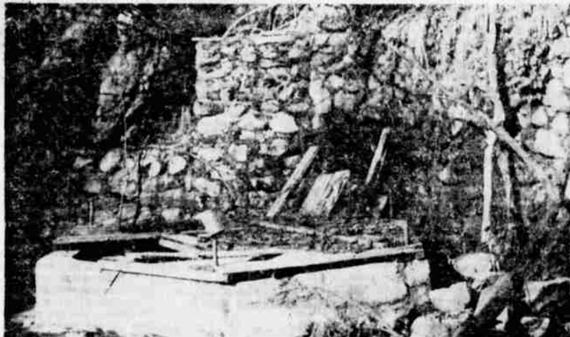
SOLID AS THE ORIGINAL ROCK is the old retaining wall at Ney Springs near Mount Shasta. It is about the only thing left intact of the once busy health resort.
