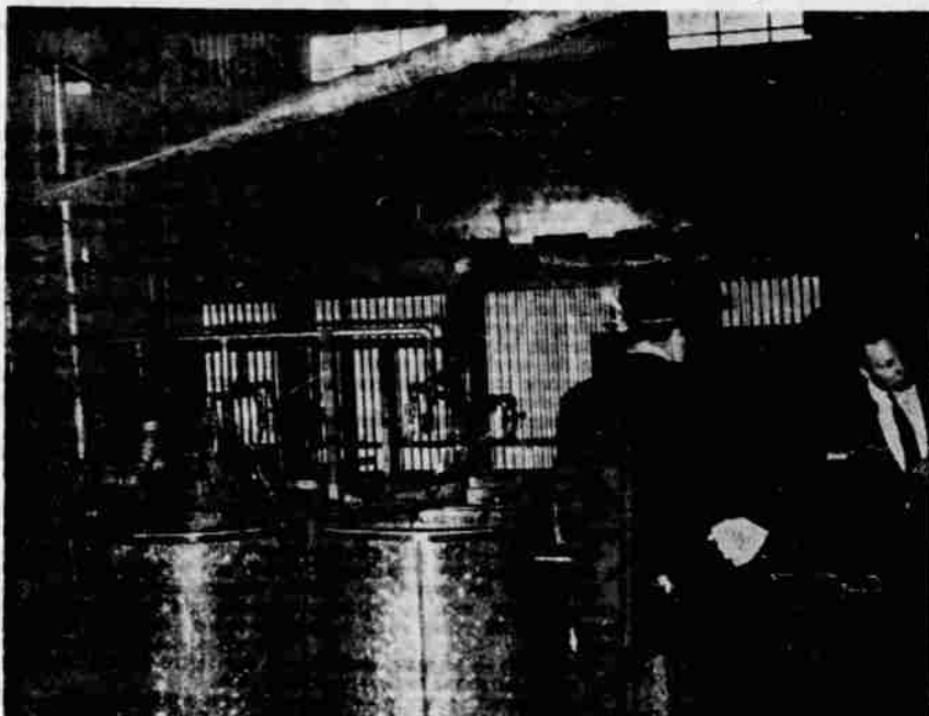
AFTER LEAVING THE PRESS the olive oil is settled in these tanks prior to filtering and further aging and canning. Wyandotte uses olives from its own growers in the manufacture of oil.
