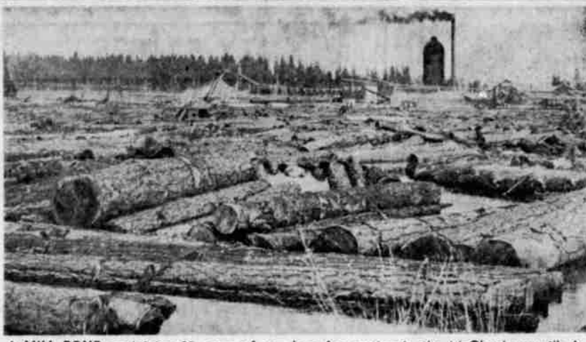
A MILL POND containing 35 acres of saw logs for cutting in the McCloud sawmills is shown here. Many of the logs shown are packaged in railroad car load lots. They are bound with steel bands and dumped in the pond. Purpose of the packaging is to preserve the quality of the timber and conserve space. Two sawmills, a power house, fuel house and fuel pile can be seen in the background.
