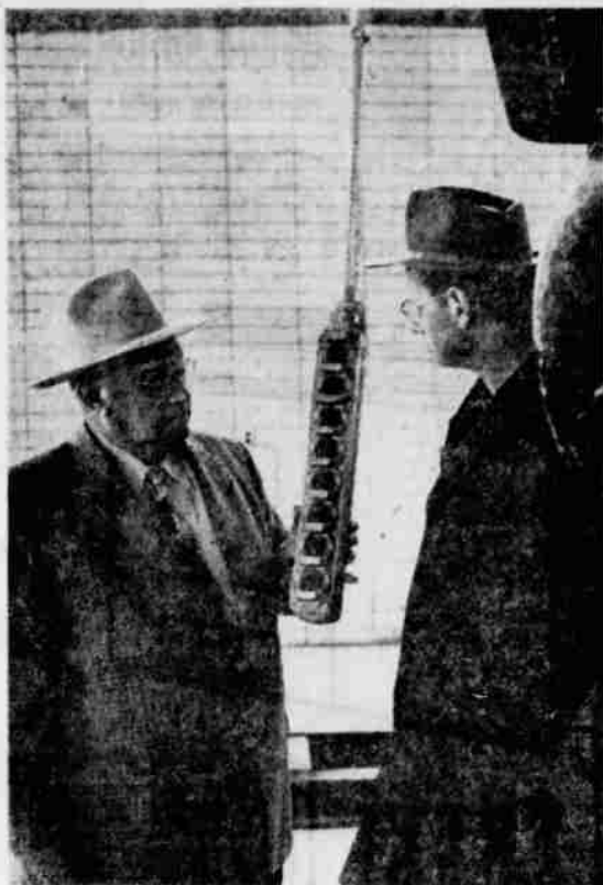
Commissioners Gowen and Frank Ganong look over the elongated control bar whose eight stops move the crane in any direction desired along the 100-ft. track. The control bar hangs within easy reach at any time.
