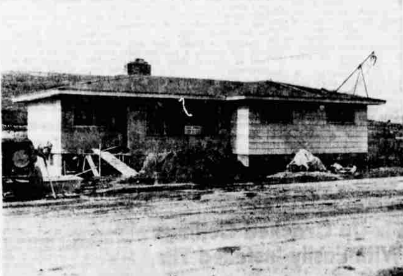
Bill Jones, who is building custom and speculative homes in West Park Addition, is one of the progressive contractors who chooses heating by Farr. This home, nearing completion, will be heated by a McPherson console forced air oil furnace installed by Farr Sheet Metal.
