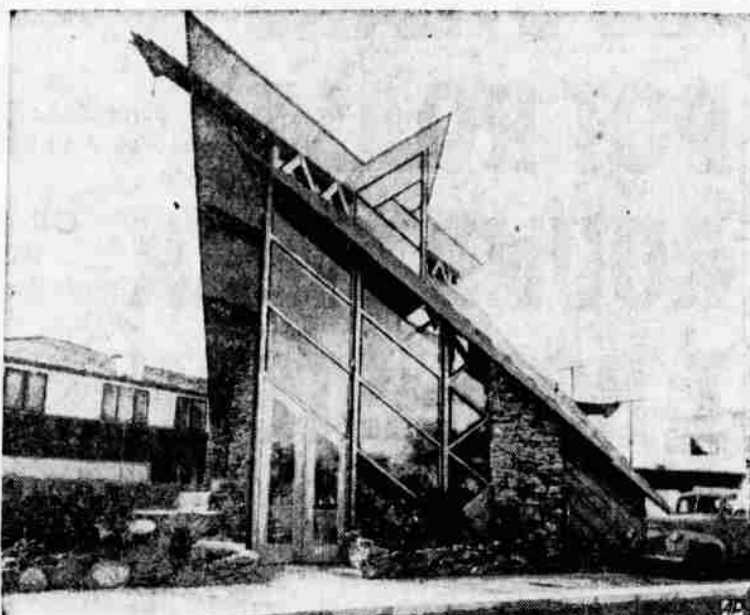
HOME WITH POINT — This angular house attracts attention near beach at San Diego, Calif. It has living room, three bedrooms and baths, a den, two kitchens, workshop, garage and boat port. Copper roof covers structure built of cedar, stone and glass.
