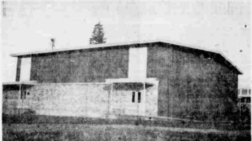
NEW MULTIPURPOSE room at Sissons Elementary School in Mount Shasta was put into service in January. The room will combine a gymnasium, band room, auditorium, basketball court and physical education classroom. The building is independent from the rest of the school. Laminated arched rafters support the roof and eliminate the need for columns. It is also virtually sound proof. George L. Ice was building supervisor for the H. Barnhart Construction Company of Medford for the $64,000 building. Howard Perrin of Klamath Falls is the architect.
