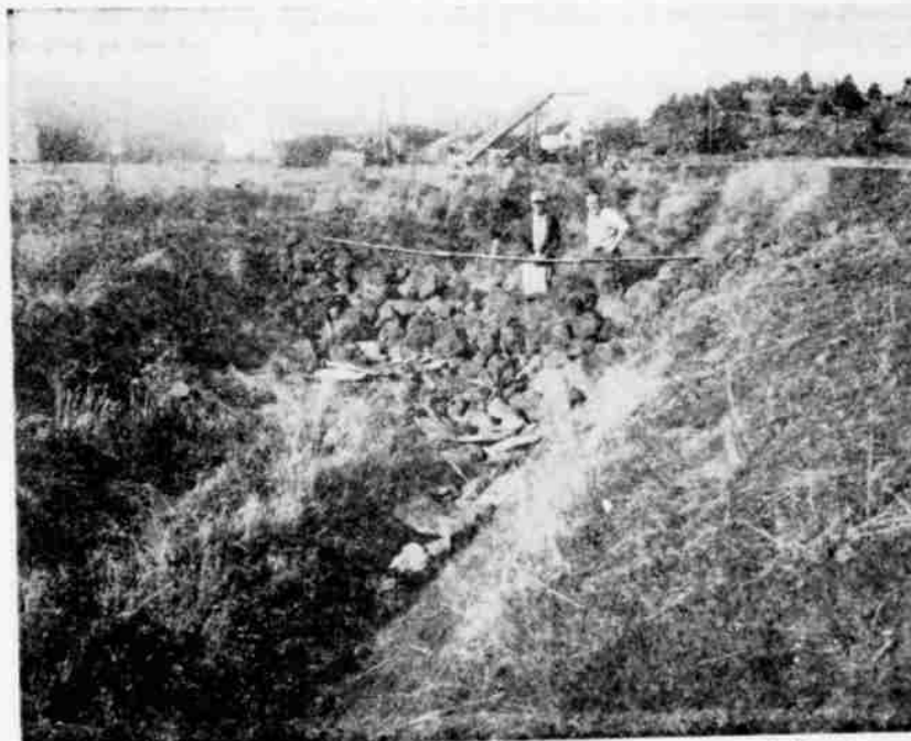
TRASH DAMS like this one on the Lee Holliday and Son ranch north of Weyerhaeuser mill are being used to stabilize ditches and gullies. The ditchbanks will be seeded with streambank wheatgrass. —Photo by Baldwin
