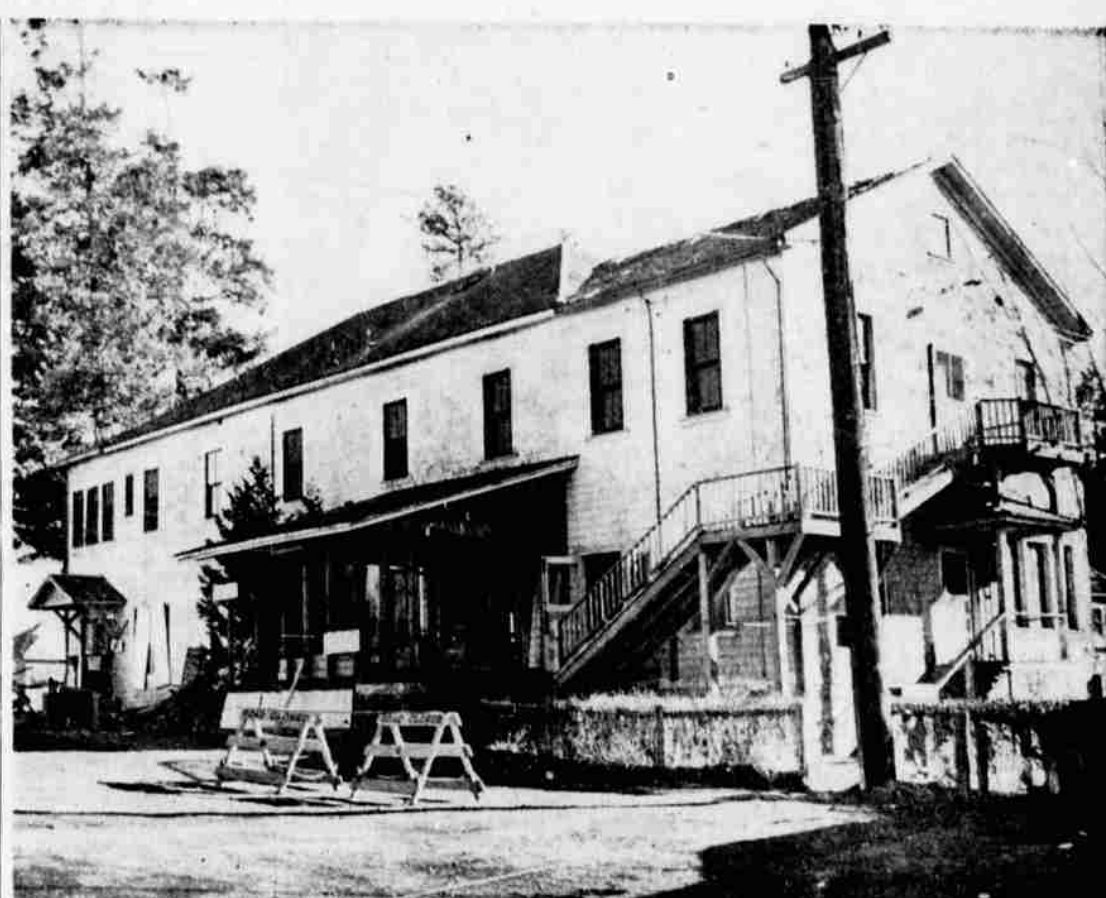
THE OLD MAKES WAY FOR THE NEW in Weed with the tearing down of the old Weed Hospital which will be replaced by a new modern medical-dental clinic, Dr. H. L. Vidricksen, M.D., Dr. V. J. Thompson, M.D., and Dr. D. L. Johnson, DDS, who have recently formed the Weed Clinic Incorporated, as the new clinic will be known, this week
