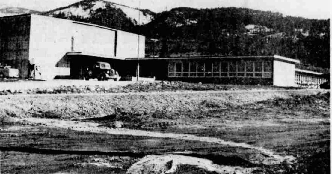
READY FOR OCCUPANCY in the fall of 1959 will be the new Mount Shasta High School building which is nearing completion. The 37,203 square foot structure, under construction by the Singleton Construction Company of Eureka, was started in May of 1958 and contains a gymnasium, class room wing and separate shop buildings. Howard Perrin of Klamath Falls is the architect for the new school which will cost in excess of $600,000. Inspector for the project is Jess E. Rodefer of Mount Shasta. — Photo by Peggy Walsh
